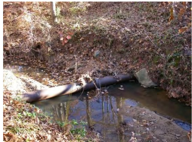
Exposed Sewer Pipe
