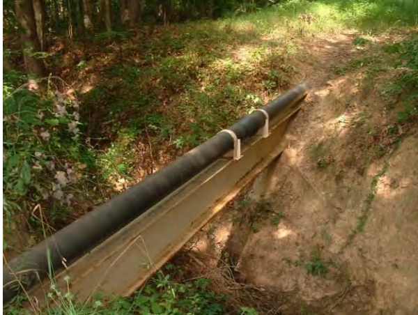
Sewer Aerial with Beam
