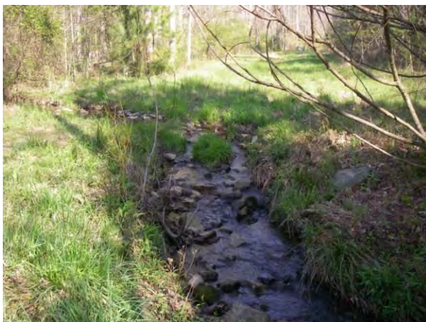
Riprap Stabilizing Easement Crossing
