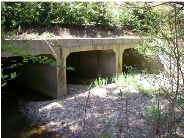
Triple Box Culvert with Sedimentation at Parkfield Drive
