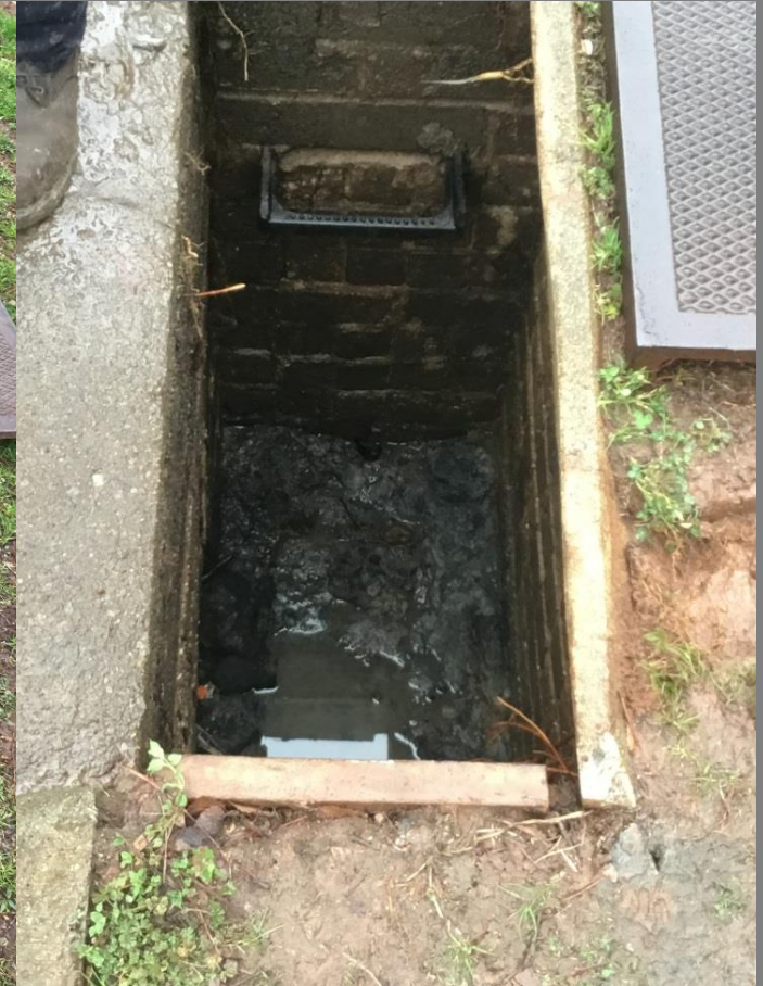
Catch basin vacuumed out
