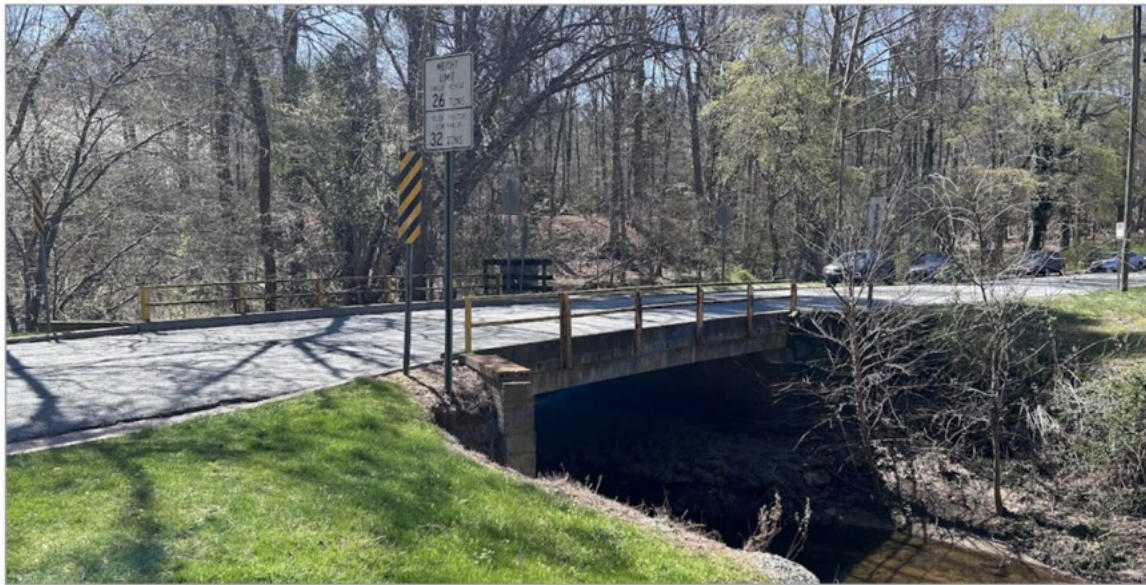
Existing Bolinwood Drive Bridge
